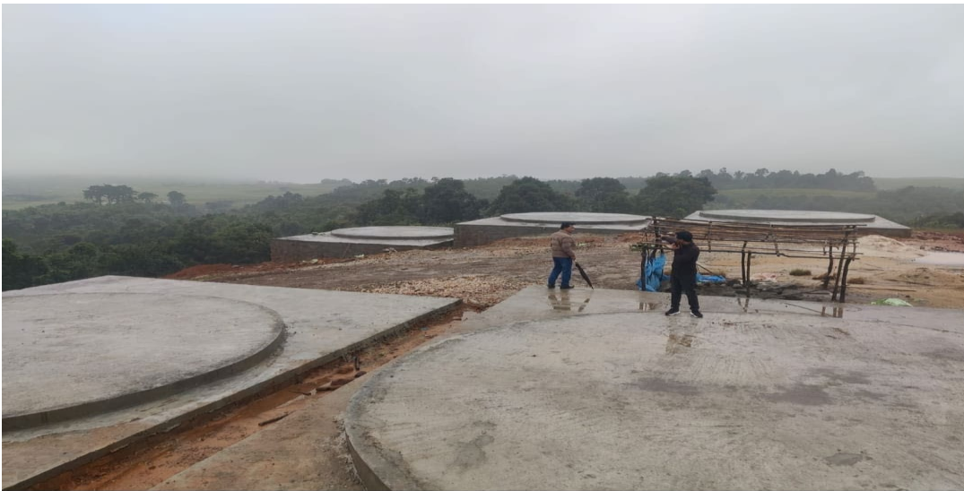
Platform Base for setting up of Yurts
